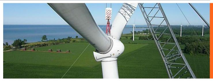
All together, the three phases of the Buffalo Atlee wind farm are located on 7 quarter sections, and will include 10 to 14 total turbines, approximately 100 to 120 m in height from the ground to the nacelle (the "hub height"), where the blades connect to the tower. The blades will each be approximately 65 to 75 metres in length, and each tower will have a generating capacity of around 3.5 to 4.5 MW.
